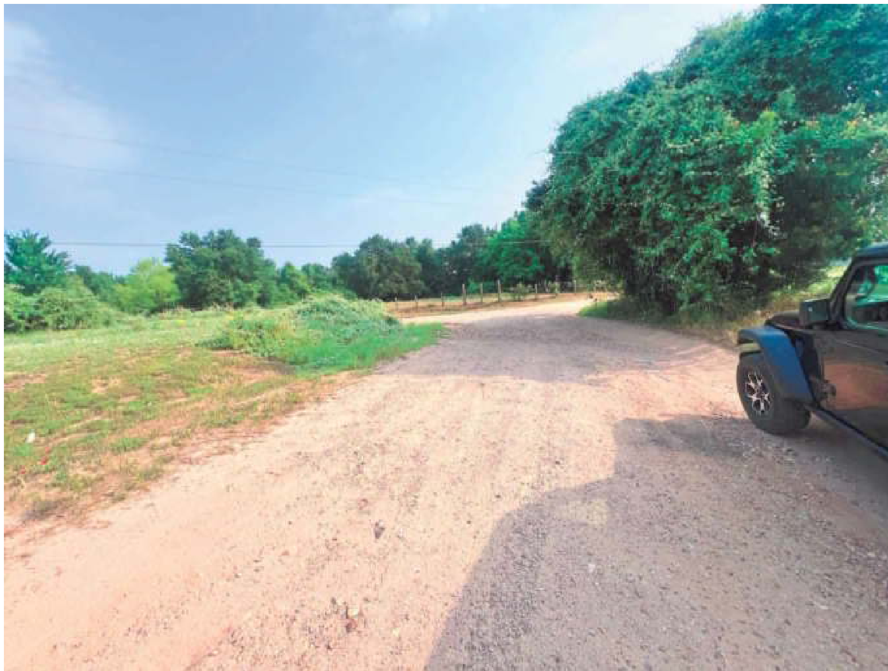
Picture 8: Looking south at the north end of the project on Elm Drive between the intersections of Oak Drive and Chestnut Drive.
