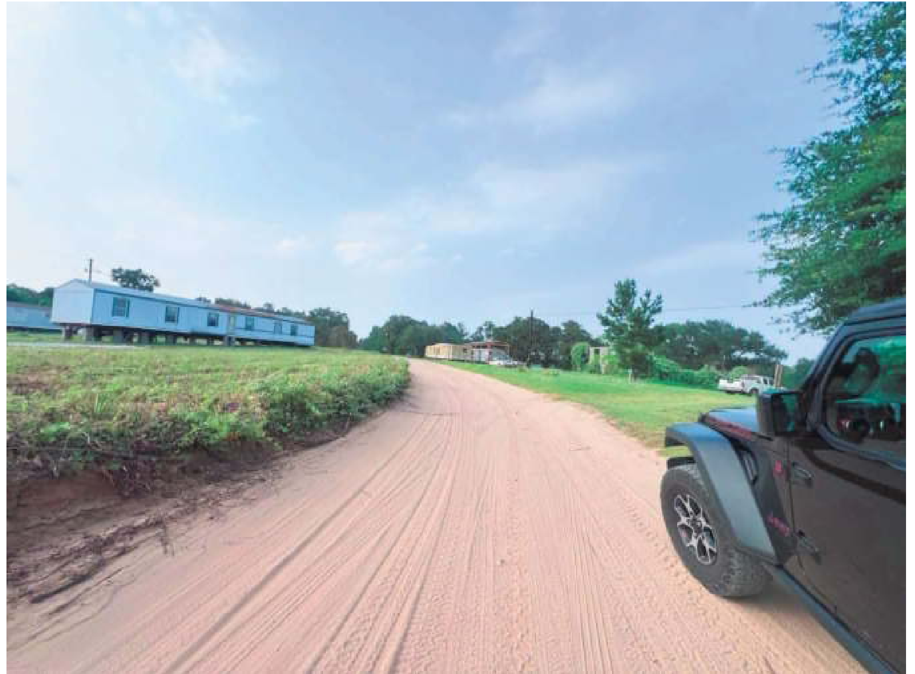
Picture 3: Looking north at the south end of the project on Elm Drive between the intersections of Oak Drive and Chestnut Drive.
